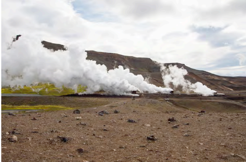
Steam rising from the geothermal power station's pipelines, Krafla, North Iceland. Photo: Lisa Paland, 2015.
