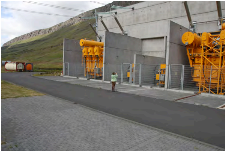
At the transformer building. Photo: Lisa Paland, 2015.
